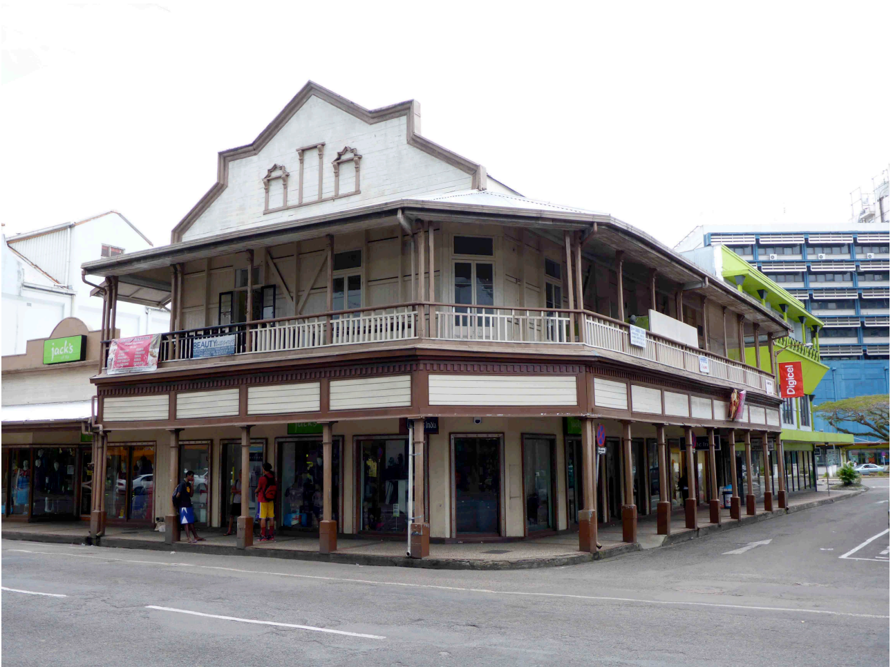
The building as it looks today, viewed across Renwick Road and looking down Pier Street. Photo courtesy Bart van Aller, 2016
